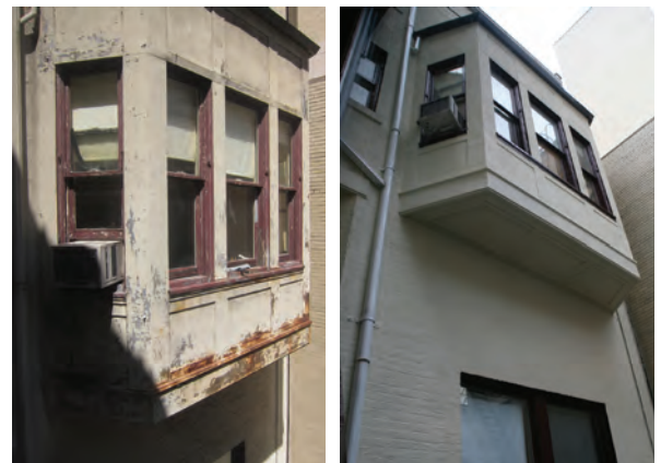
Restoration of the KF House
